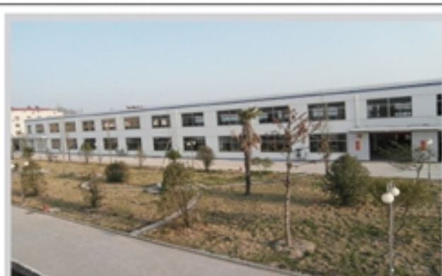
Factory Building 厂房厂区
